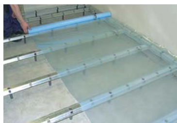
Installation, floating 22 mm chipboard
